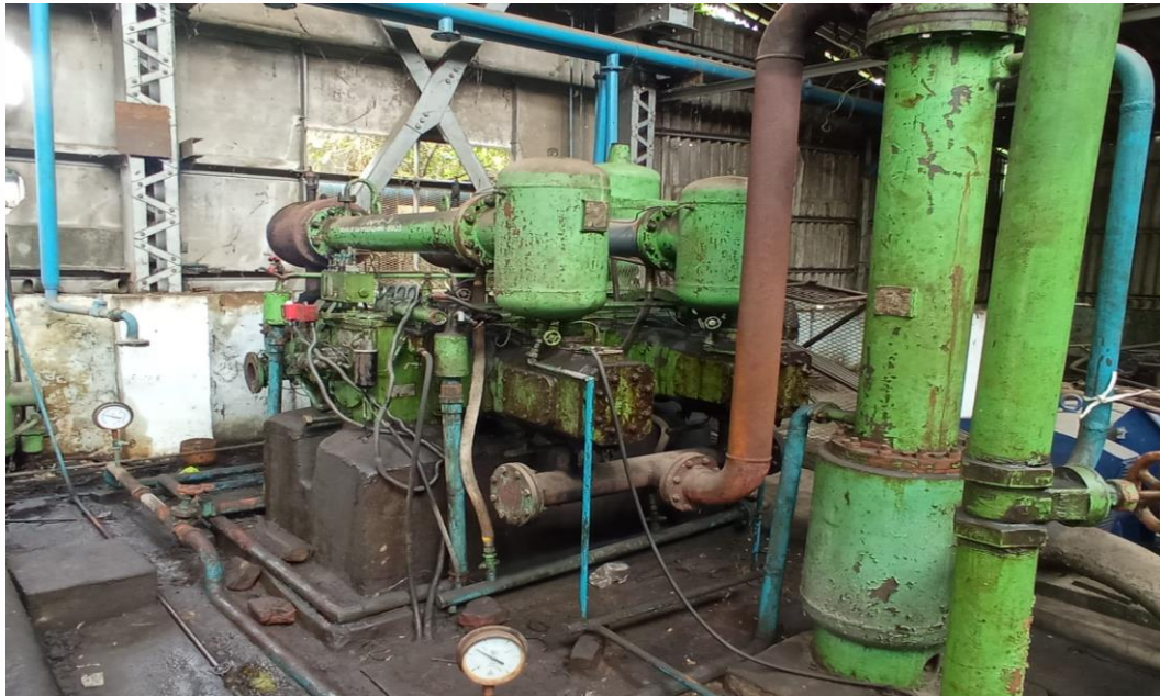
Replacement of Reciprocating Compressor
